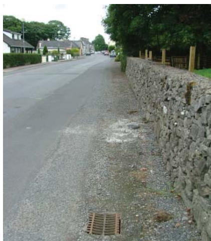
Photo 18: Footpaths are generally only found on one side of the street, except in the village core.
