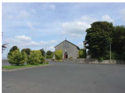
Photo 19: Church car park.
