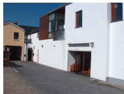
Photo's 24, 25 & 26: Good modern design of shop fronts co-existing with traditional, Belmullet, Co. Mayo.
