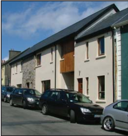
Photo 31: Very successful modern infill building - this broad infill site has been successfully sub-divided - through various design elements, notably the subtle recess and projection of the facade with the use of different materials such as stone, plaster render and timber. A modern fenestration pattern and windows design also maintains and reinforces the traditional vertical emphasis of the streetscape, as does the alternation of roof heights.
