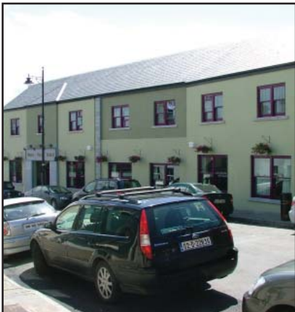
Photo 32: The use of different shades of colour, together with subtle recessions, projections and deflections of the facade assists in integrating this hotel development into the streetscape. These features echo the traditional plot division and 'urbangrain' of the streetscape.
