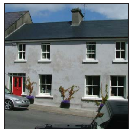
Photo 36: This is a nicely refurbished townhouse on Chapel Street. Although it is not refurbished to strict conservation principles - it is more than acceptable. Ground floor windows and door openings are broader than those typically found in the traditional streetscape, yet they retain an adequate recess, deep cills, and a vertical emphasis with two-over-two timber sash windows - all very complimentary.
