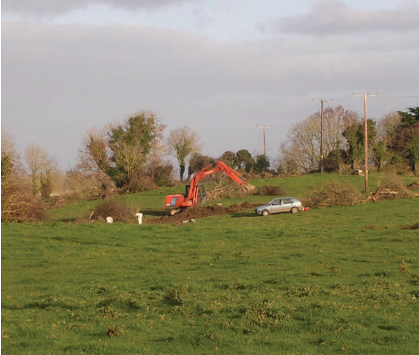
Hedgerows being removed
