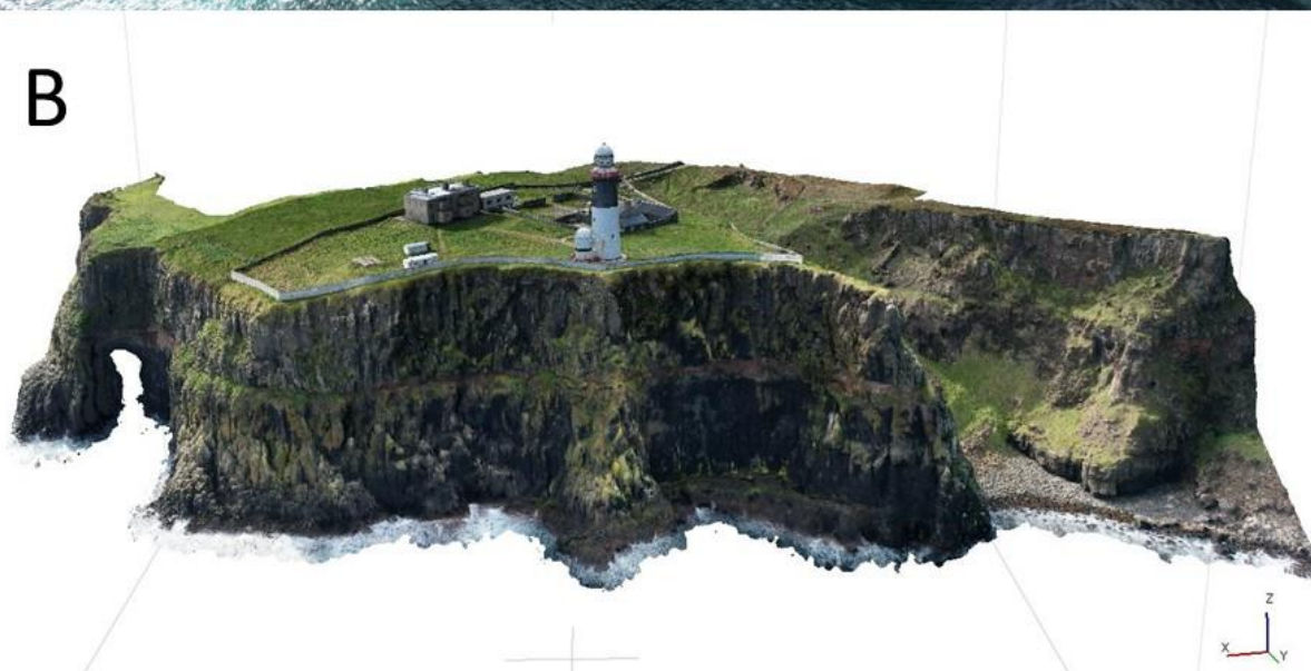
Figure 18: A comparison of the East Lighthouse on Rathlin Island as seen by (A) drone and (B) the SfM based digital model
