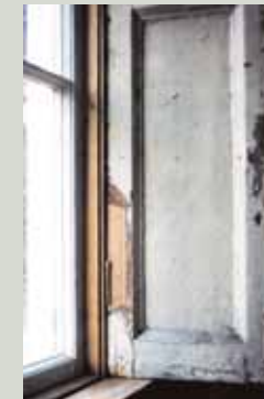
A cabinetmaker carried out some repairs to this shutter. The illustration shows new timber pieced in at the lower hinge, where decay had taken place, prior to repainting the timberwork
