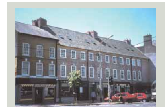
This restored terrace of early eighteenth-century houses retains the original appearance of the fully visible sash frames, which is quite different to the later house on the left
