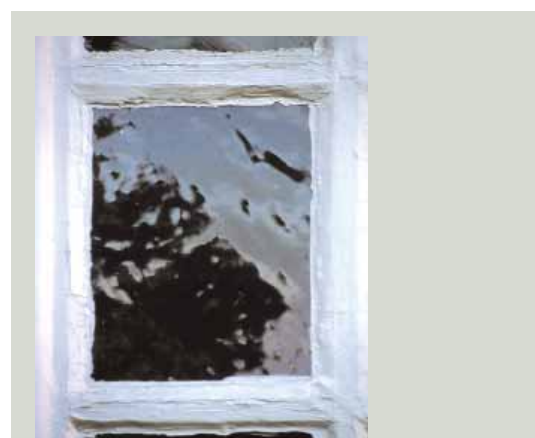
Early cylinder glass has an extremely hammered looking surface and is quite speckled with bubbles or seeds, like the pane in this early eighteenth-century window
