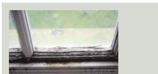
This mid eighteenth-century oak sash was dipped before being repaired with new parts. The ultimate effect of the chemical on the oak is obvious and serious: the original fabric is now incapable of repair
