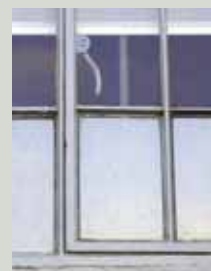
The mastic should be a smooth bead and must be fully sealed to prevent moisture attacking the steel, as was done in this maintenance project
