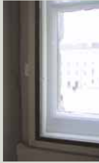
A double-glazed internal casement panel has been fitted to this sash window. The design is such that there is little or no visual impact from the exterior. Given the wide panel frame, this design would not be appropriate in a location which contains an authentic period interior. The opening in this case did not have any shutters or other internal joinery
