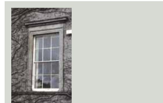
The sash window shown here was installed in about the 1780s (it is now freshly glazed with new cylinder glass). Extremely thin glazing bars like these were made possible by using a metal core to strengthen the bars. Joinery standards improved generally towards the end of the eighteenth century to keep up with this new fashion for slimly profiled windows
