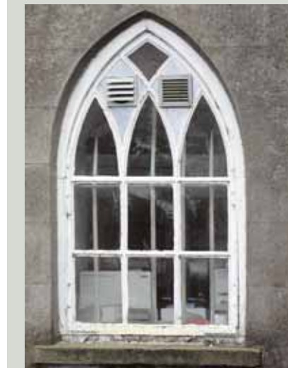
In a historic building, vents should be sited in locations where they do not require invasive structural work and so that they are unobtrusive. They should never be placed in historic windows like this unusual eighteenth-century casement, whether or not historic glass would be affected
