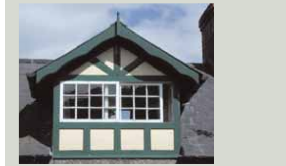
One side of a horizontal sliding window (sometimes called a Yorkshire sash) can be pushed open, while the other is fixed shut
