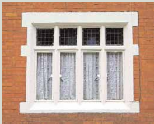
The original catches and stays survive on these metal casements. They should be retained and cared for whenever the window is undergoing maintenance, as they are an integral part of the original window
