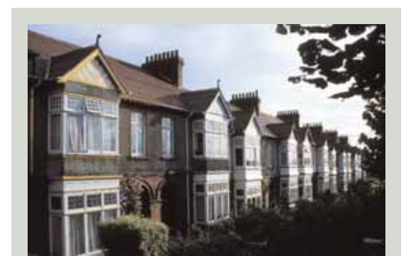
This terrace of thirteen houses was built in 1907. Almost all retain their original windows of stocky timber casements which contain decorative toplights
