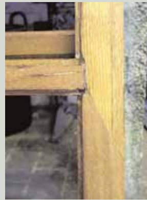
This oak sash has been repaired with new timber scarfed in, which matches the grain density and direction of the original. The repair is of high quality and should last indefinitely
