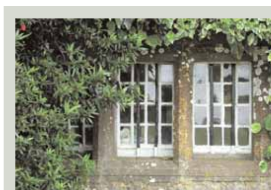
Lead-glazed fixed lights and casement windows of the seventeenth century are extremely rare in Ireland. Called 'quarry glazing', lead panels were still being made into the early eighteenth century, but were seen as inferior to timber-framed windows in every way
