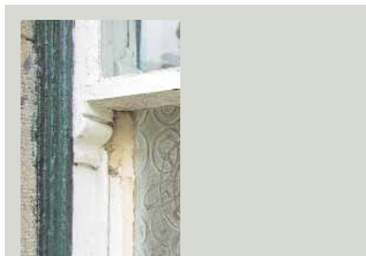
An early twentieth-century horn or joggle. The more slender the timber in a sash, the weaker the important joint at the meeting rail of the top sash, which bears all the weight of the sash as it hangs closed in position. Letting the 'horn' remain at this joint after construction, and decoratively shaping it, was a practical response to strengthen this vital joint. Generally, the smaller and plainer, the earlier the horn. More elongated and curvilinear shapes became common in the late nineteenth century
