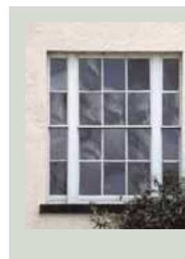
Historic glass types have a different appearance to modern float glass. They are wavy, often tinted or speckled and have a softer sheen. The presence of historic glass gives an irreplaceable visual quality to the appearance of an old window
