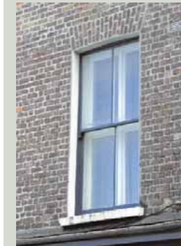
Complaints about draughts are nothing new. 'It is pitiful to see the extent to which women, and men too, allow themselves to be dominated by a little wind and a little weather... They must seal themselves up hermetically by weather-strips, and thus exclude the little sweetness that would make its way to them', reported the Irish Builder in 1888. This bulky internal window must reduce indoor light a good deal as well as reducing natural air flow
