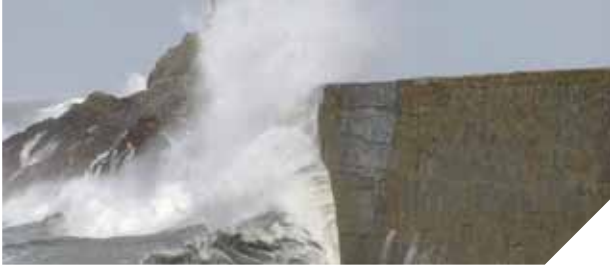
Artificial breakwaters in San Vicente, Galicia (Spain)
