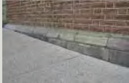
Access ramps against the façade of a building can conflict with or obscure important architectural features such as stone plinths. While a ramp may be physically separated from the masonry by a barrier to allow its removal without damage, the visual impact still needs to be resolved
