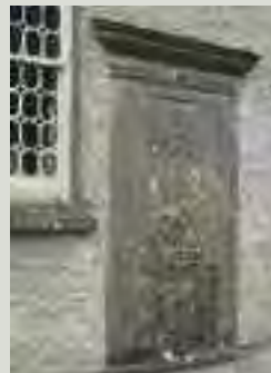
Carved stone plaques are found most often on the walls of public buildings such as schools and churches – as with this wall monument – but many domestic buildings also have datestones. Whether or not the structure has changed use or the carving is now illegible, efforts should be made to retain interesting plaques or monuments in situ
