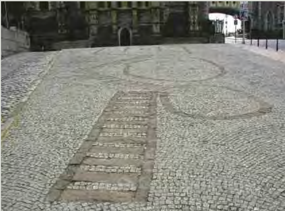
Where new paving is required, the opportunity may arise to have a pavement designed especially to suit the character of the area. This paving outlines the site of excavated Viking housing and is interspersed with inset bronze plaques depicting finds made during archaeological excavations in the area
