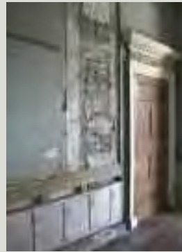
Later finishes or features may cover earlier elements of interest such as this sixteenth-century doorway, partly covered by re-used original panelling and an eighteenth-century doorcase; it may be necessary simply to record the earlier feature while retaining the high-quality later work in place undisturbed
