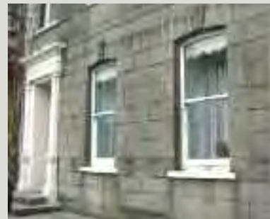
Render is a traditional coating which contributes both to the weathering performance and appearance of a structure. This house has been partially faced in Roman cement in imitation of rusticated ashlar and, while not the original finish, clearly contributes to its character
