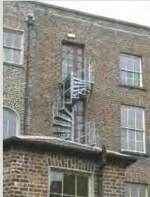
Proposals that require the conversion of original window openings into doors to facilitate escape will require very careful consideration and should avoid impacting on surviving early or original windows and on important elevations. There may also be a potential impact on nearby windows which may require re-glazing with fire resistant glass
