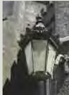
Exterior fixtures and features vary widely in size, function and materials. Some, such as the lead gas lamp illustrated here, have been adapted to electric light and continue in use. But, even where redundant, such fixtures and features are often important to the character of a structure or area, in addition to being well-crafted items in themselves
