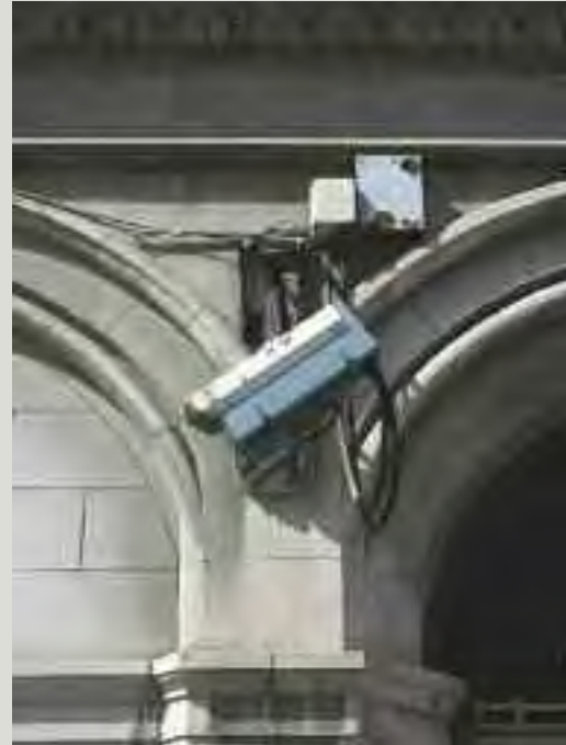
Fixtures or features fitted without thought as to their visual impact can adversely affect the character of a structure or area. The removal – or resiting – of such items should be encouraged whenever possible. The method of fixing should be reversible and, on stone or brick façades in particular, made into existing joints rather than through the masonry to avoid scarring
