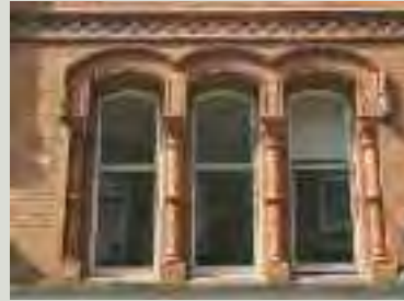
The treatment of structural openings may add considerably to the character of a building; here the elaborate brick and terracotta detailing and the arched window-heads add architectural distinction to the opening
