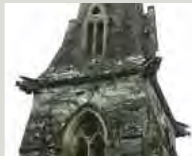
Masonry details associated with roofs may be functional or not. Whether they are plain or decoratively detailed, they add character to a roof and, even if now redundant, should be retained
