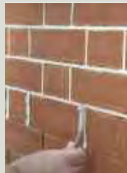
Where the repointing of historic brickwork is proposed, the specification of the mortar and the style of work to be used in repointing should be provided. Where specialist work will be required such as wiggling and tucking, demonstrated here, the work should be undertaken by experienced personnel
