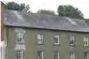
The removal of chimney stacks can damage the appearance of an entire building
