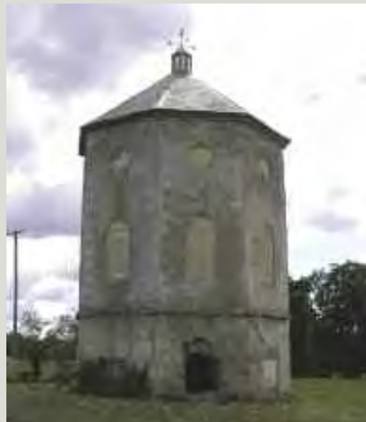
The original roof of this eighteenth-century dovecote was lost; however sufficient evidence survived to design a new roof which complements the structure
