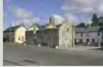
In this instance, a ruined market house marks the centre of a planned village. Despite its ruined state it forms a local landmark which, if lost, would remove the focus of the historic townscape
