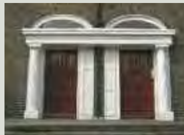
The inaccurately-detailed alteration of doorcases or other features will, in most cases, be to the detriment of the structure and often affect the character of an ACA also
