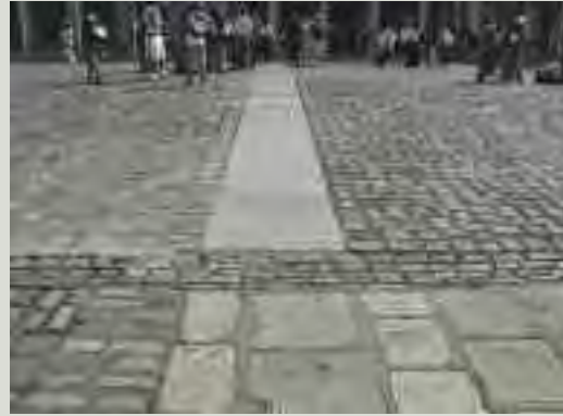
Traditional surfaces finishes can cause problems for those in wheelchairs or with walking difficulties but accessible routes can be provided through these areas using complementary materials
