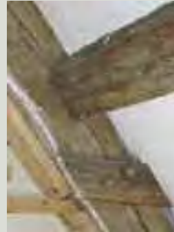
The structural components of a roof may contribute to its character. Here a seventeenth-century pegged oak roof structure survives largely intact, with the carpenter's numbers visible on some timbers
