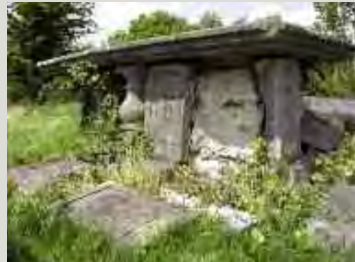
While there is generally a respect in communities for burial grounds, the wish to maintain them should not lead to over-enthusiastic or misguided 'tidying-up' works or the uninformed reconstruction of damaged memorials. Where repairs are planned to damaged memorials, all fragments should be identified and reset using an appropriate mortar, and any poorly executed previous repairs rectified, if this can be achieved without further damage. Specialist advice will usually be required
