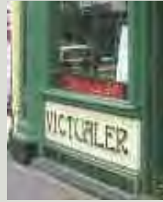
The functional and decorative features common to many historic shopfronts including tiled stall risers (top), ornate brackets (middle) or original shutters (bottom) are all part of the special interest of a shopfront
