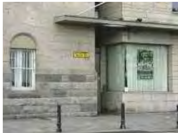
A planning authority should promote good standards of conservation in development works to the protected structures in their ownership. This example shows the junction between a successful modern addition and the original local authority building
