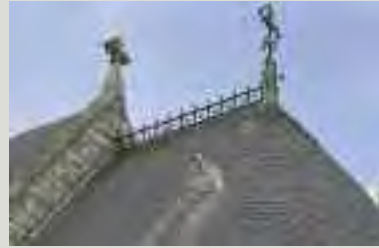
Ridge tiles, finials, iron cresting and weathervanes are found on many structures and give a building its distinctive outline against the sky. Repairs should follow best practice for each particular material
