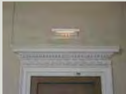
The use of standard signage may not be appropriate in high-quality interiors. Alternative designs are available which minimise the visual impact while fulfilling fire-safety obligations
