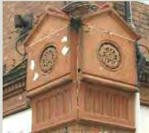
Materials such as terracotta and faïence tend to be very durable. However, they can be damaged by aggressive cleaning methods. In this case, a later paint finish, together with the original fireskin of the terracotta, have been removed, exposing mortar repairs and old defects and leaving the ceramic vulnerable to future accelerated weathering
