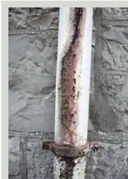
Iron rainwater goods such as gutters, hopper heads and downpipes are extremely long-lasting if given regular and frequent painting to prevent corrosion. Where they have already started to rust, the iron should be properly prepared before repainting
