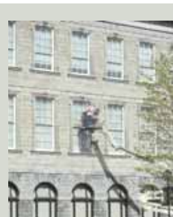
Specialised equipment such as cherry-pickers may be needed to allow inspection of the upper levels of taller buildings
