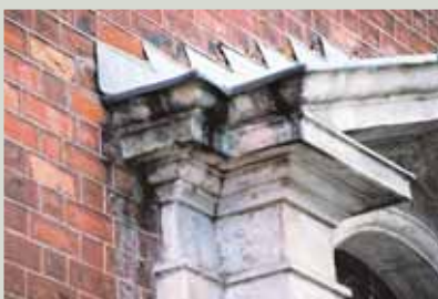
It may sometimes be necessary to add flashings where none originally existed if it is clear that damage is being done
