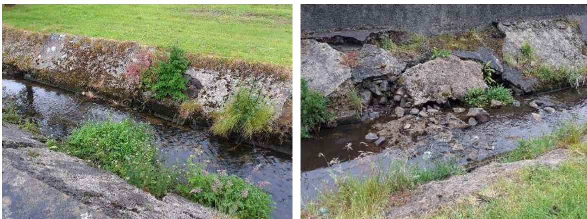
Plate 86: The stream along Marian Row, showing some areas of streamside vegetation and areas where the concrete bank has fractured
