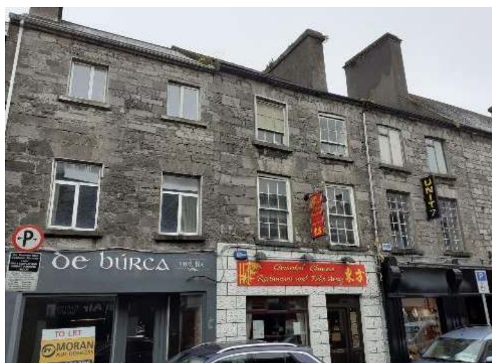
Plate 76: Some buildings on Main Street in Castlebar have attractive stonework
