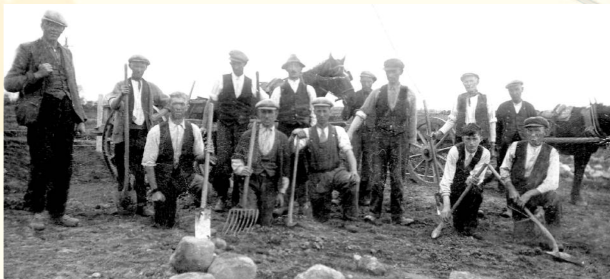
There was great excitement in Brickens in September 1940 when a group of local men were employed by Mayo County Council to tar the road through the village. Pictured are ganger Dick O'Gara with workmen Thomas Kelly, Michael Healy, Michael Carney, Kevin McHugh, John Brady, Billy Lohan, Michael Kirrane, John Connelly, Luke Morley, Tom Lyons, Mike Morley and Paddy Murray. Picture: Western People Archive
