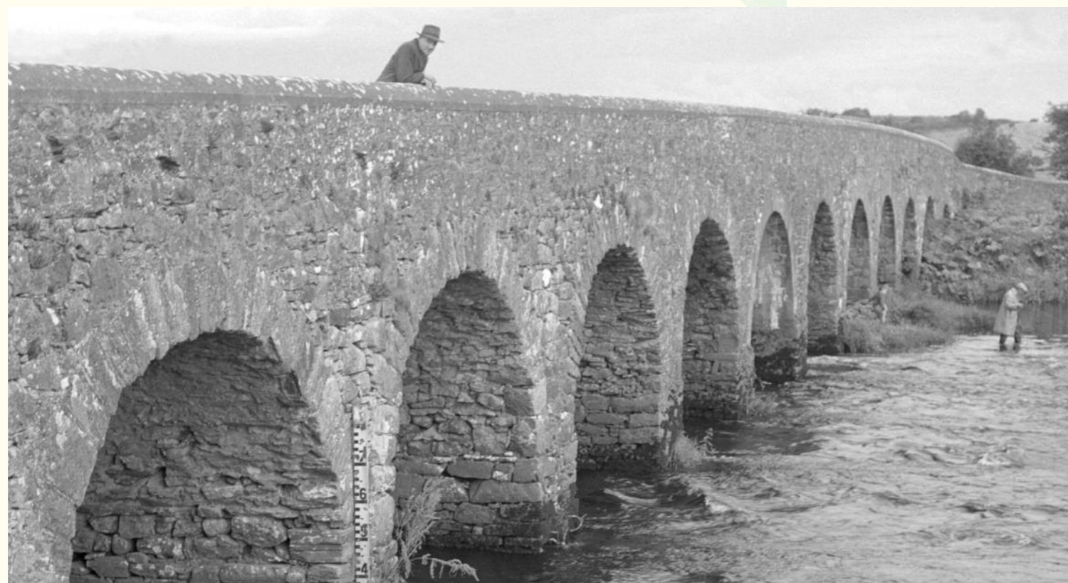
The old Ballylahan bridge pictured in 1960 before being replaced with the current bridge. Picture: Western People Archives
