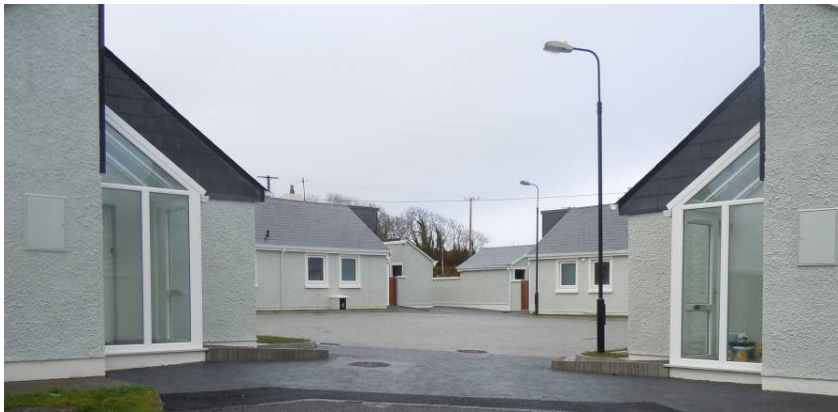
Energy Efficiency Programme: Sea View Place, Ballycastle Upgrading of BER to houses including energy efficient heating systems, replacement windows & doors, new porches & external hard landscaping
