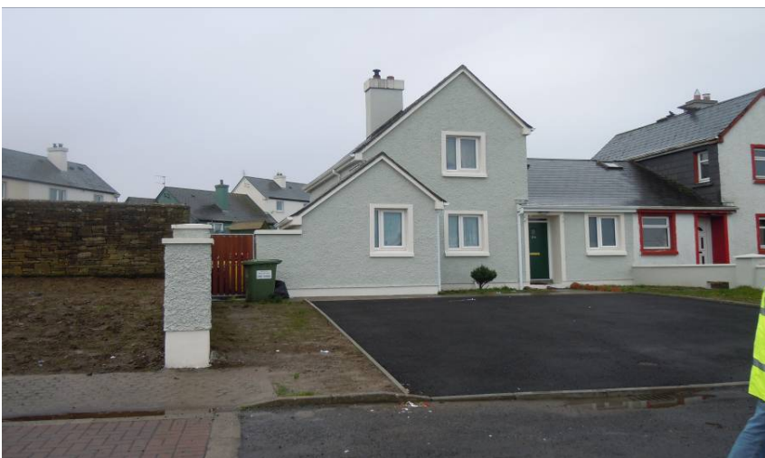
The Enhancemnt works (EEP) undertaken in Sea-View, Ballycastle now complete
