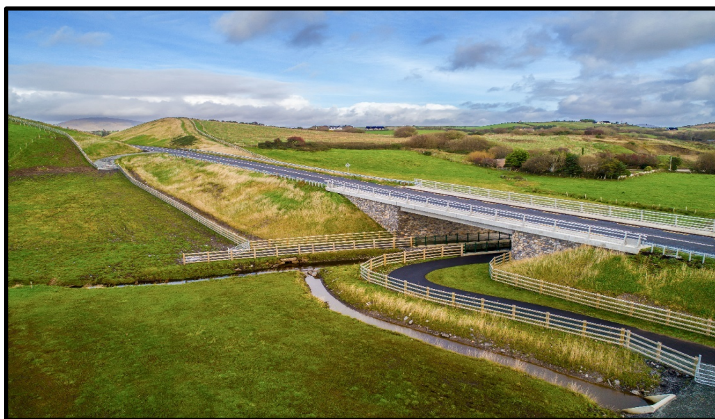
N59 Rosow Bridge
