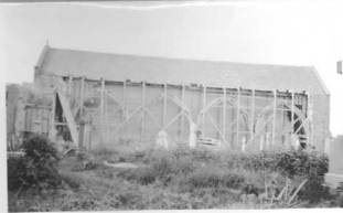
WORK OF RECONSTRUCTION IN PROGRESS, 12th JUNE, 1937.
