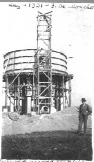
Reservoir nearing completion Reservoir nearing completion 1931
