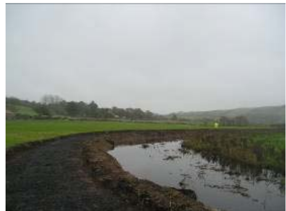
Clearance and drainage at Aitreech,
