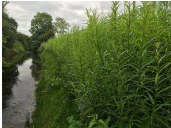
Image of works 3 months after completion
