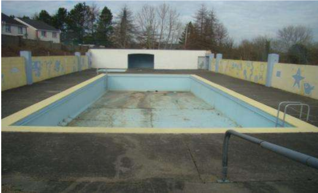
Existing Pool prior to refurbishment.
