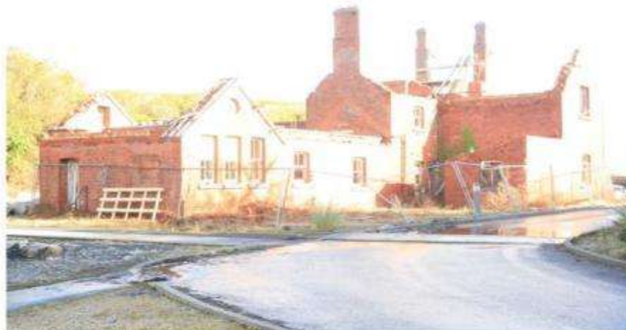
View to rear of building (facing N-E) prior to reconstruction works – February 2016
