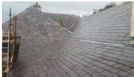
Ballinrobe House: Roof Repairs
