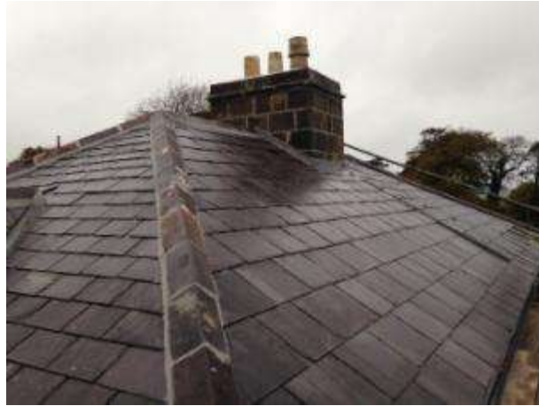
Ballysakeery Glebe House: After
