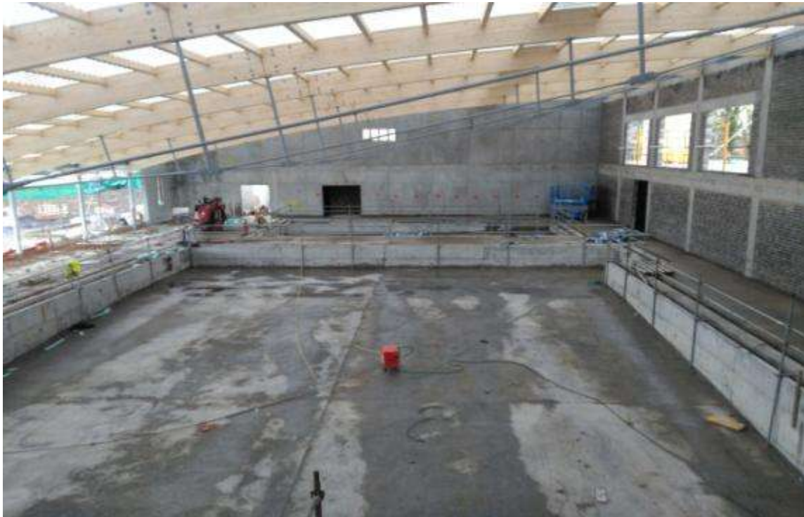
Refurbishment Works to the Charlestown Outdoor Swimming Pool.
