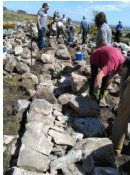
Repairing Stone Walls on the Greenway
