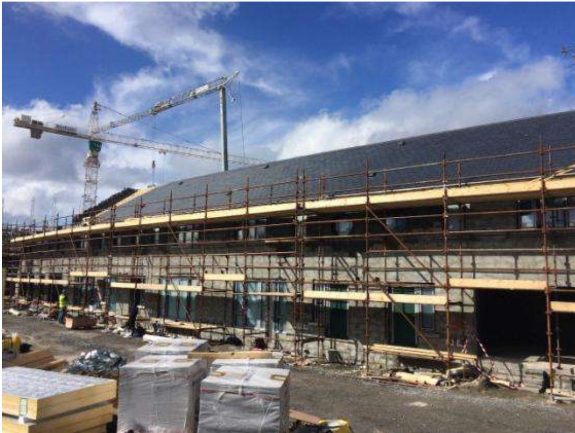
Progress of works to date on site in Tubberhill.
