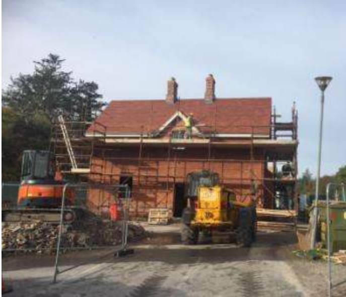
Greenway Activities Services Centre under construction
