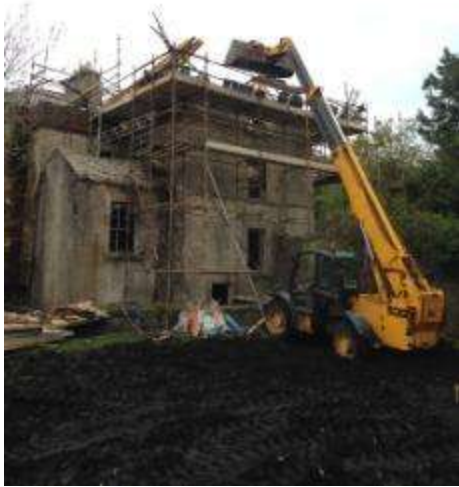
Ballysakeery Glebe House: Before
