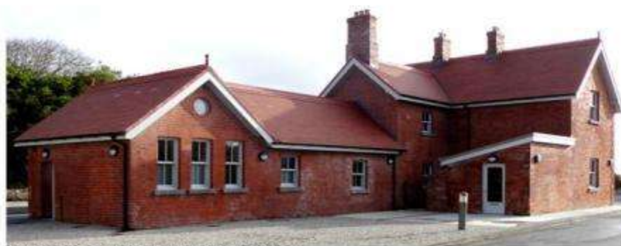
View to rear of building (facing N-E) post completion – March 2017
