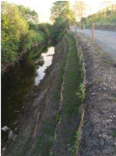
Just after Construction
