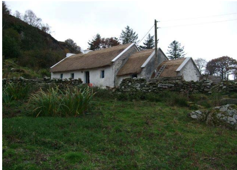
House Re-Thatch & Refurbish – Knappagh, Westport.
