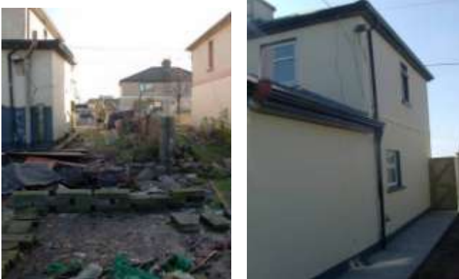
Housing Refurbishment Programme - Before and after
