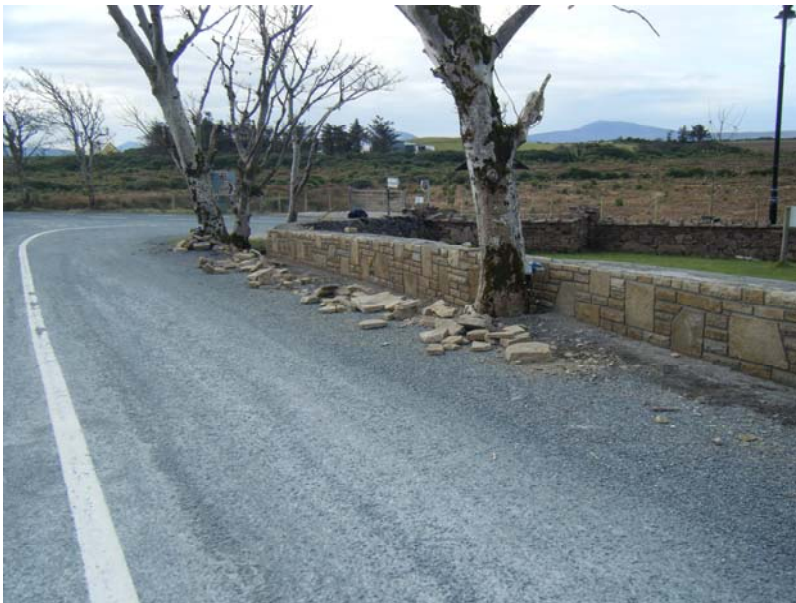
New wall construction in the village of Ballycroy.
