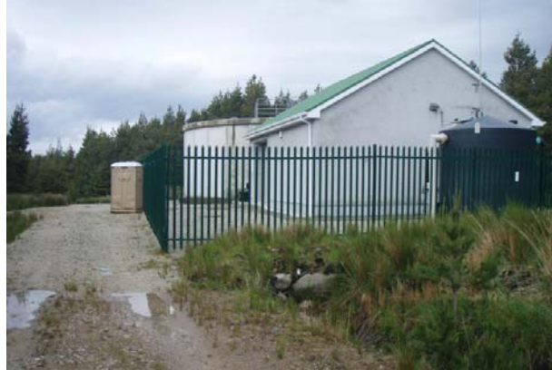
Ballycroy Group Water Scheme Treatment Plant.
