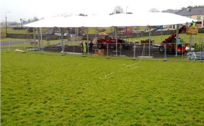
Ballyhaunis Multi Use Games Area – Under construction
