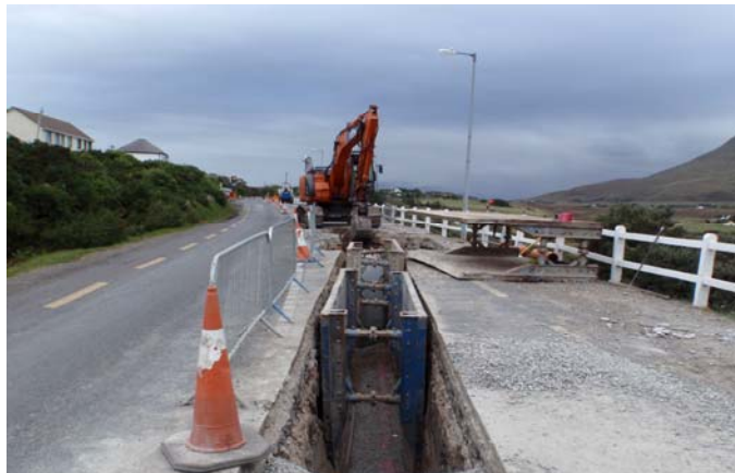
Achill Sound Sewerage Scheme
