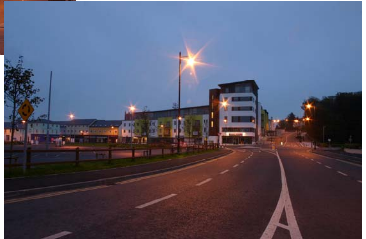
New Road at Mountain View, Castlebar
