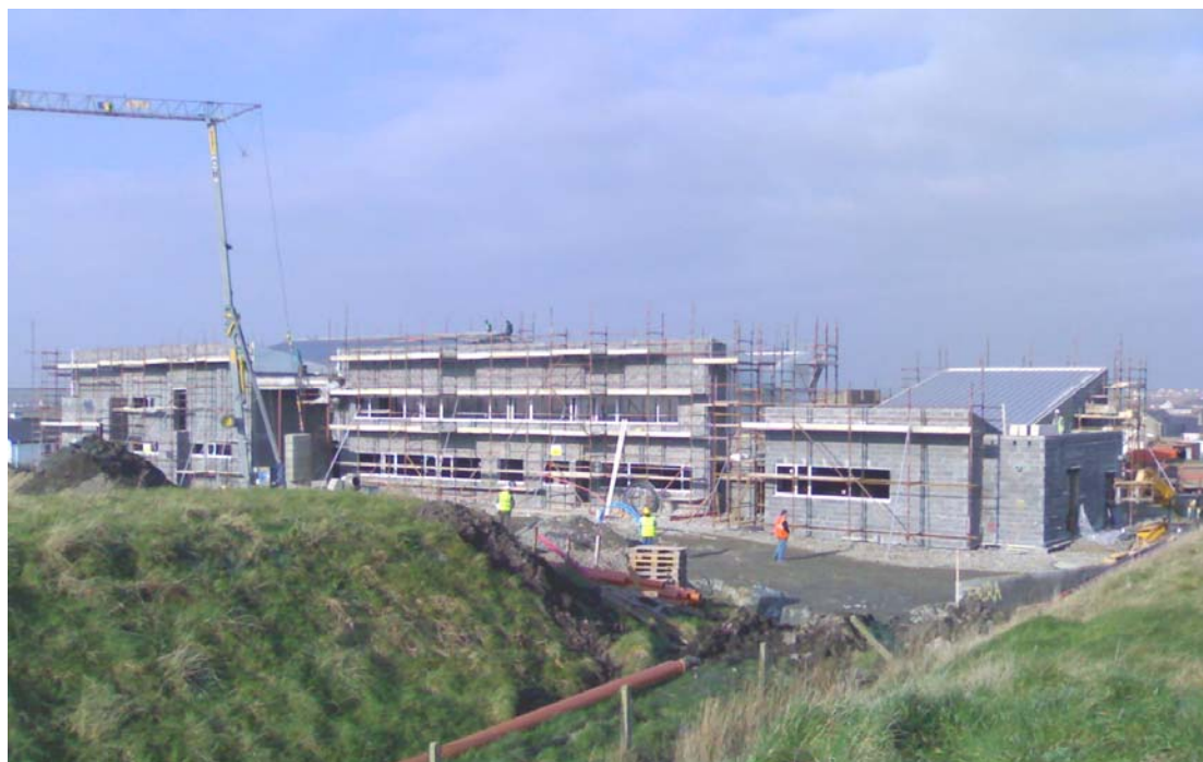
Works in progress on the new Belmullet Civic Centre.
