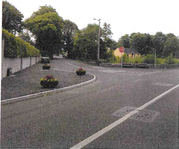
Realigned and improved junction Quay/Creggs Road.
