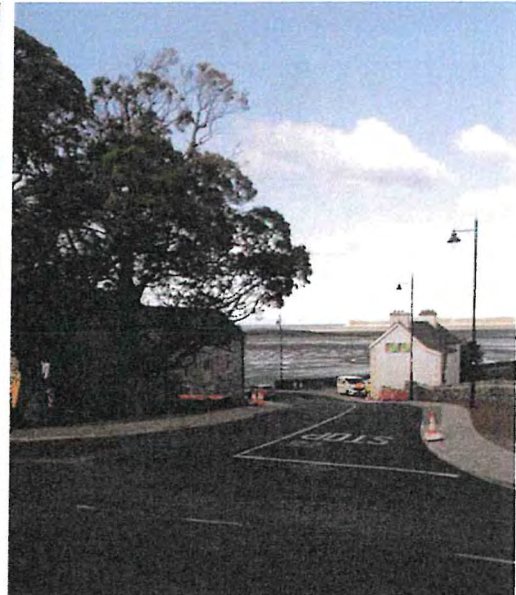
Realignment of the R314/L5191 junction at Killala completed in April 2019
