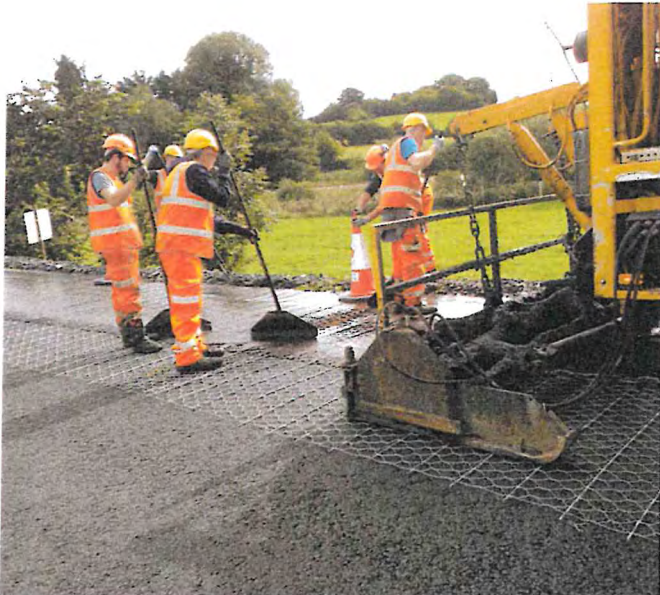
Mesh reinforcement and strengthening of R310 Regional Road at Rehins, Ballina.
