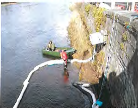
The Council was involved in the clean-up of an oil spill on the river Moy which necessitated the placing of a boom in the water to contain it together with all day monitoring to ensure it remained in place.
