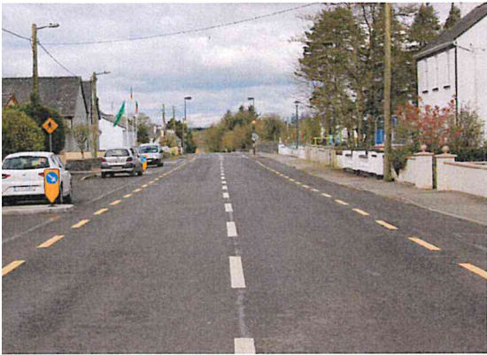
Restoration Improvement Works at Irishtown R328
