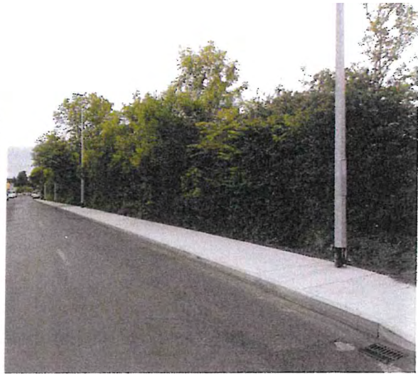
Behy road extension of Public lighting & footpath.
