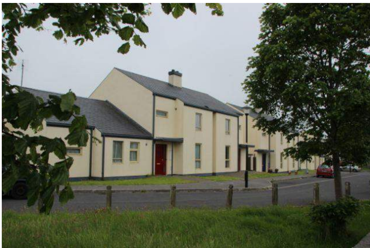
Ongoing local authority housing maintenance
