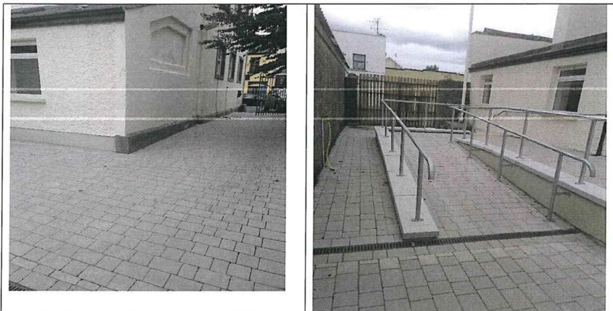
New entrances at Court House, Swinford constructed with funding from Redz.
