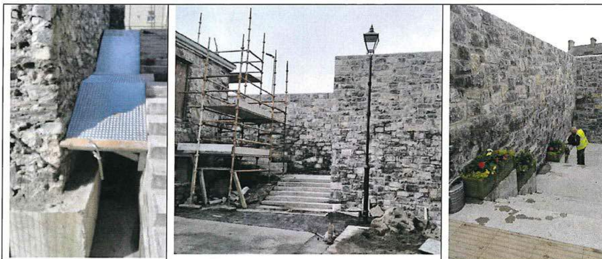
Works at O'Rahilly St
