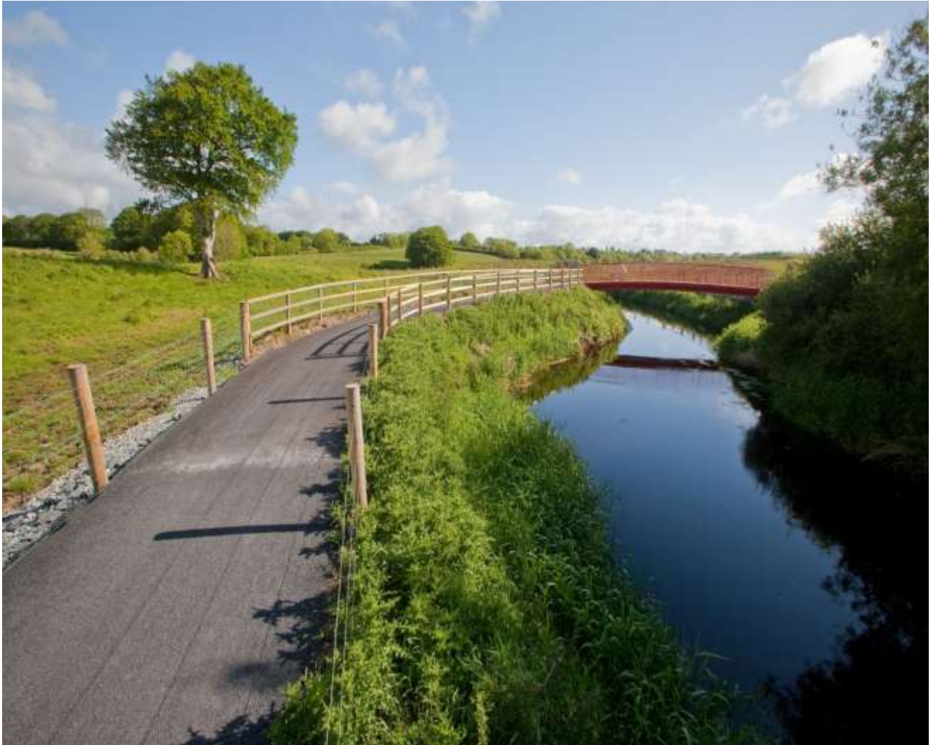
Castlebar to Turlough Greenway
