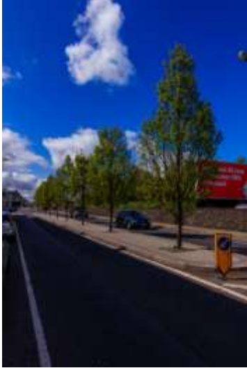
Kevin Barry St, Ballina - New road Island with trees completed in 2014.
