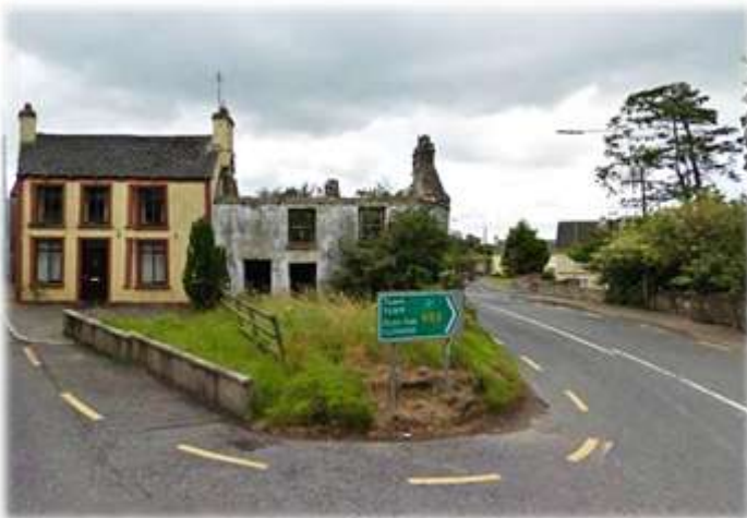
Devlis Junction Before Construction
