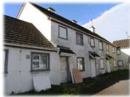
Parkview Prior to / and after Works
