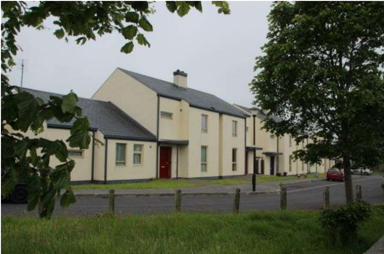
Ongoing local authority housing maintenance
