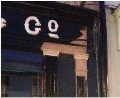
Repairs, Moran & Co. Westport
