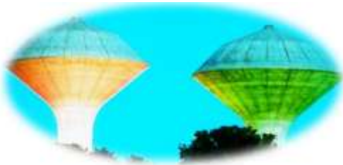
Ballinrobe Water Towers
