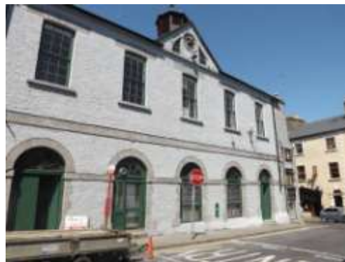
Former Ballinrobe Courthouse: After
