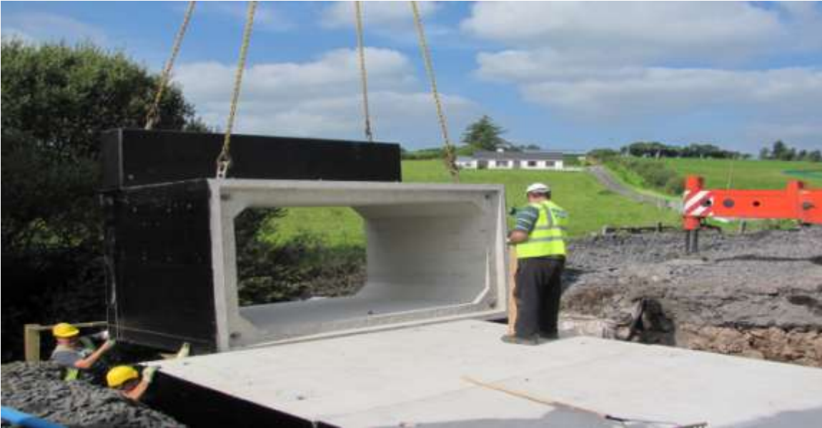
Cummer Bridge, Glenisland, Castlebar. (R312)
