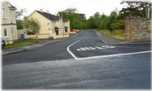
Esker Pines (Before and After)
