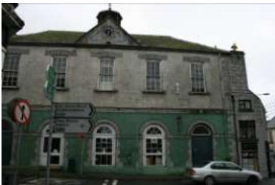
Former Ballinrobe Courthouse: Before
