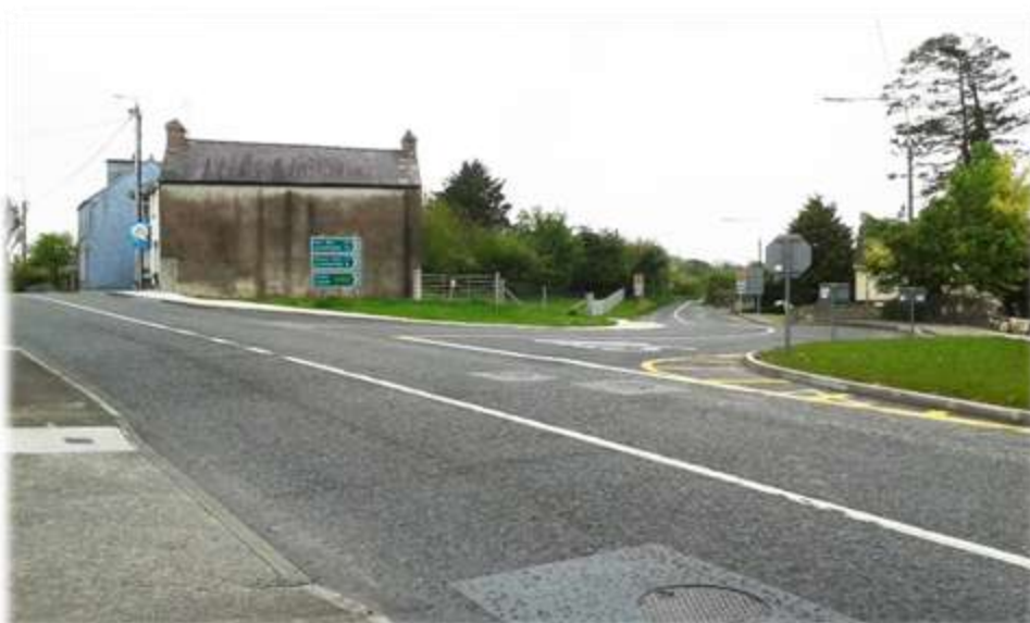
Devlis Junction After Construction
