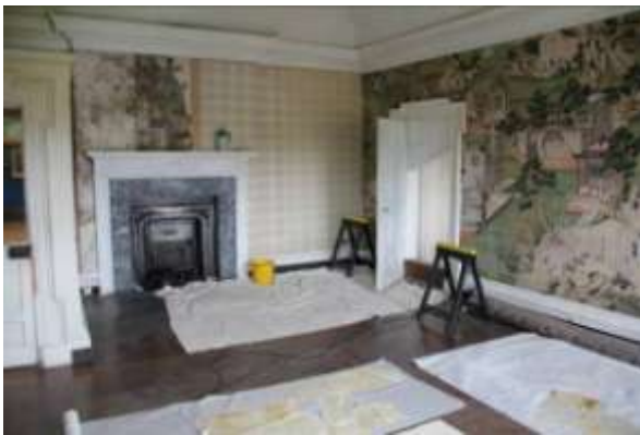
Repairs to Chinese wallpaper, Westport House
