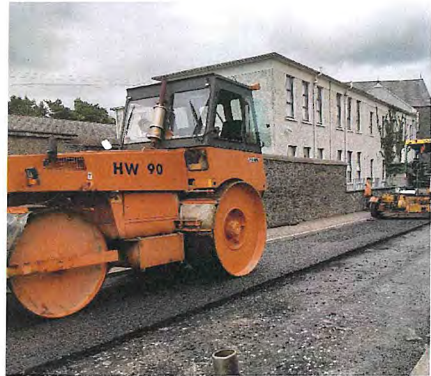
Hot Rolled Asphalt works at Convent Hill, Ballina.
