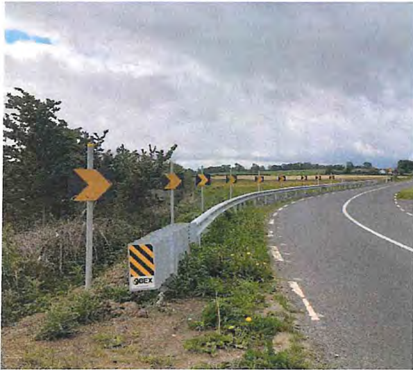
Vehicle restraint system installed R310 near Rehins
