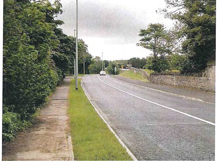
R315 Road Realignment and additional Public Lighting South of Killala
