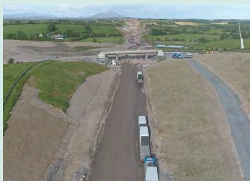
N5 Project: Islandeady Bridge Works
