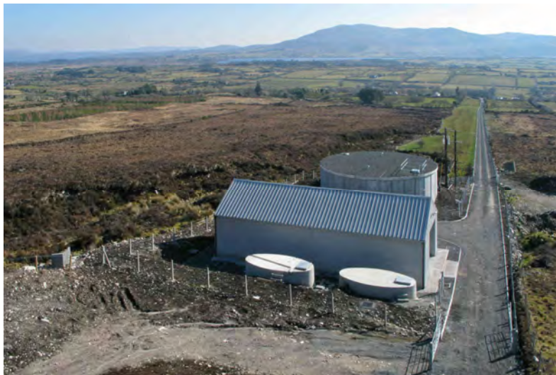
Nephin Valley Treatment Plant
