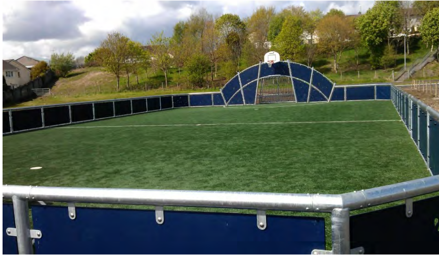
Newly completed Multi-Use Games Area in the Town Park, Castlebar.
