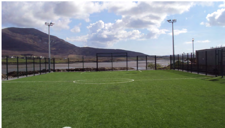
Newly completed Multi-Use Games Area in Pollranny .
