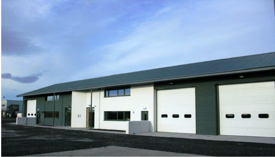
The newly completed 'Moneen Depot' welfare facility, in Castlebar.
