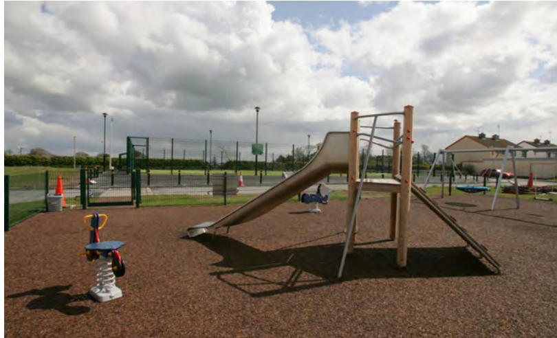
Newly completed Playground Area in Ballinrobe .
