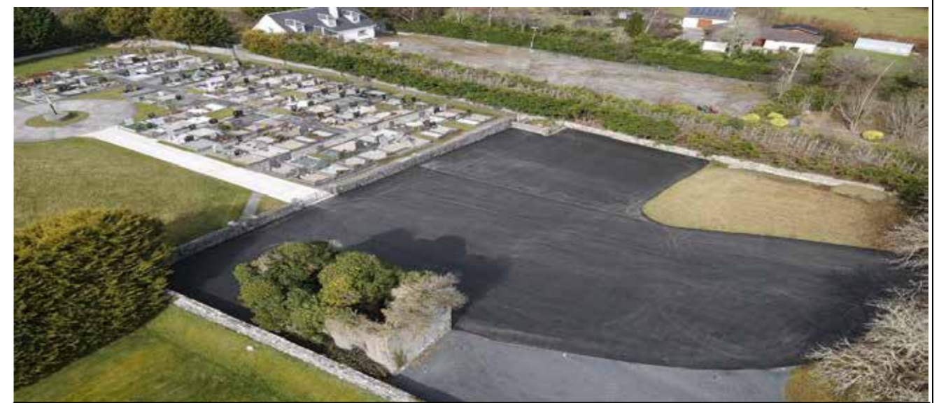
Resurfacing Works – Cong Burial Ground Car Park
