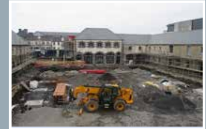
Works progressing at the Ballina Innovation Quarter.
