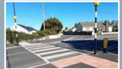
New Pedestrian Crossing at Crossmolina.
