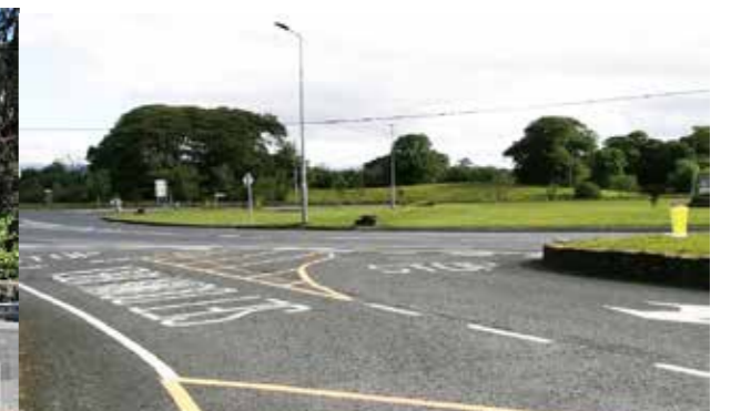
Road Realignment and Landscaping at Bohola
