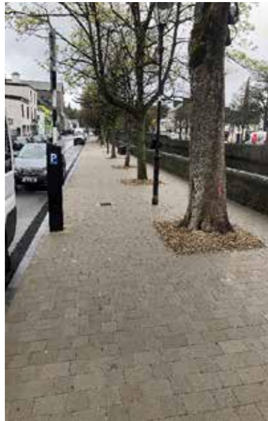
Paving of the South East Mall in Westport Town
