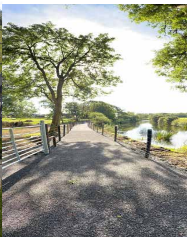
Upgrade and Extension of Bowers Walk Ballinrobe
