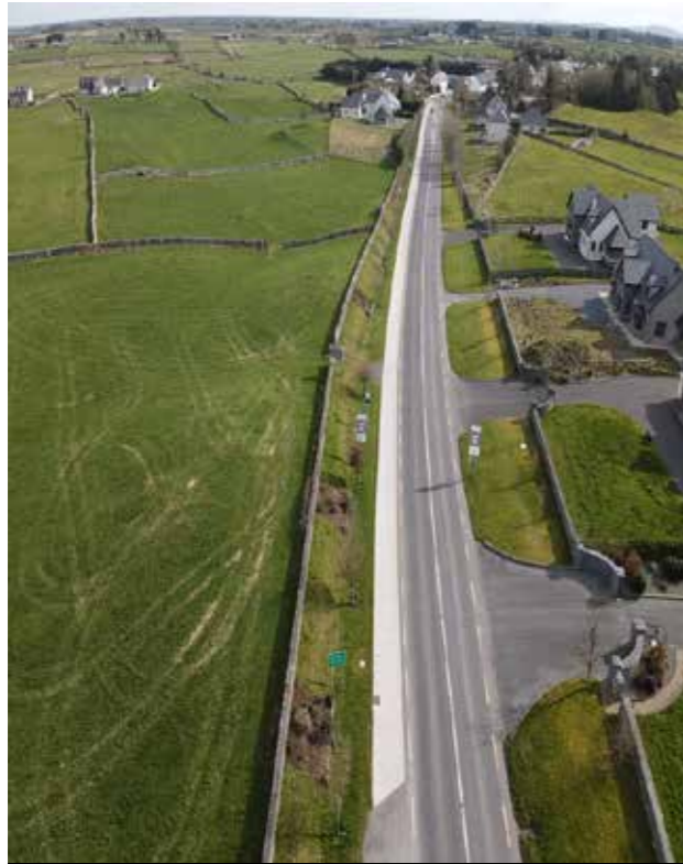
Extension of footpath Kilmaine
