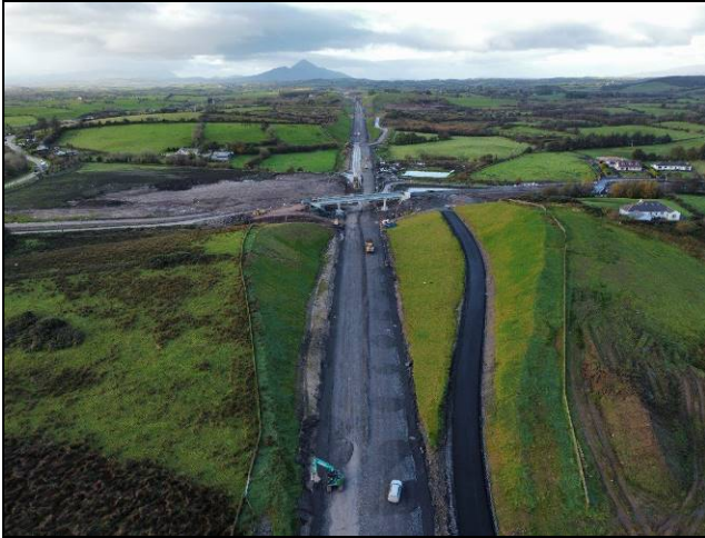
N5 Westport to Turlough Road Project-Works at Islandeady Road
