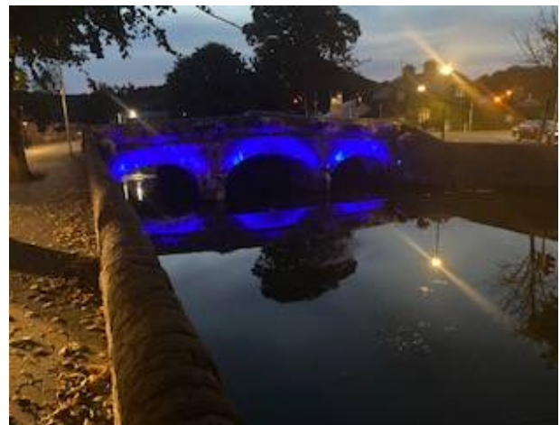
Bridge over Carrowbeg River, Westport on World Drowning Prevention Day
