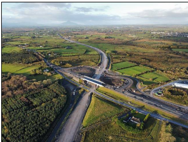
N5/N84 Grade Separated Junction
