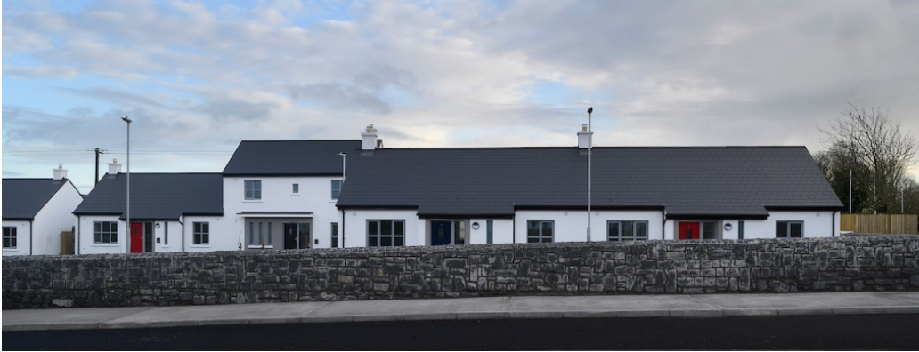
Recently Completed Parke Housing Scheme
