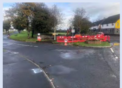
Pedestrian Crossing works at Crossmolina.
