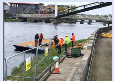
Repair Works to the Salmon Weir Pedestrian Bridge
