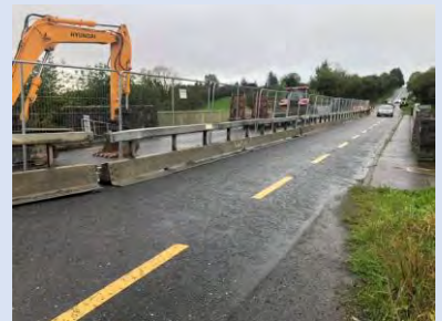
Works at Knockadine Bridge, Crossmolina.
