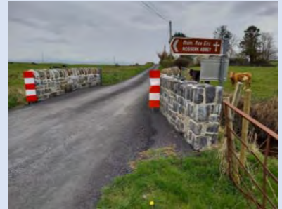
Rosserk Bridge & Surface Dressing works.
