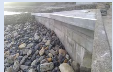
New wave wall at Kilcummin Harbour
