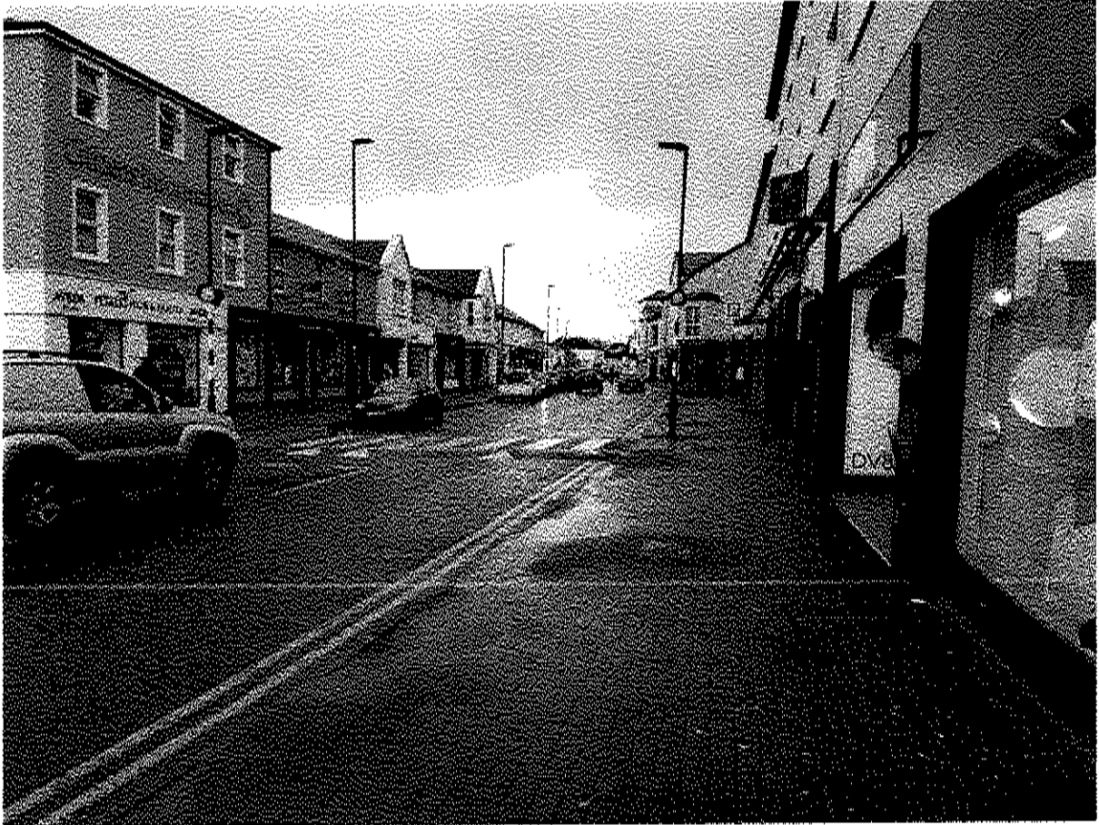
Hopkins Road Enhancement, Castlebar
