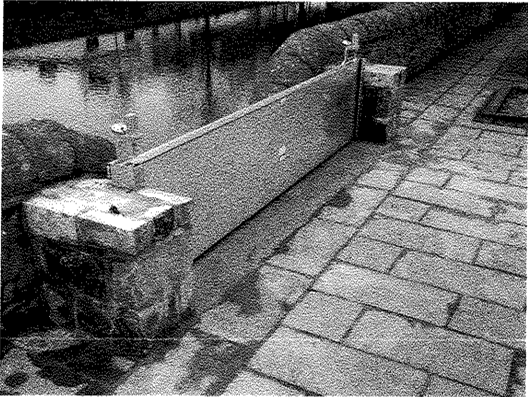
North and South mall flood gates
