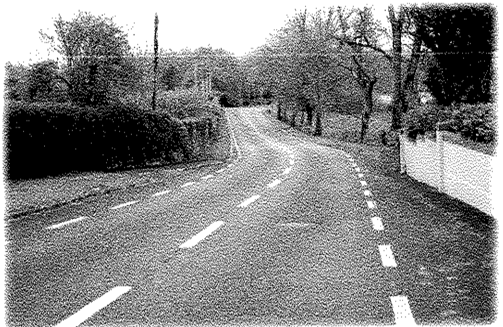
Completed pavement strengthening works taken from The Neale Junction
