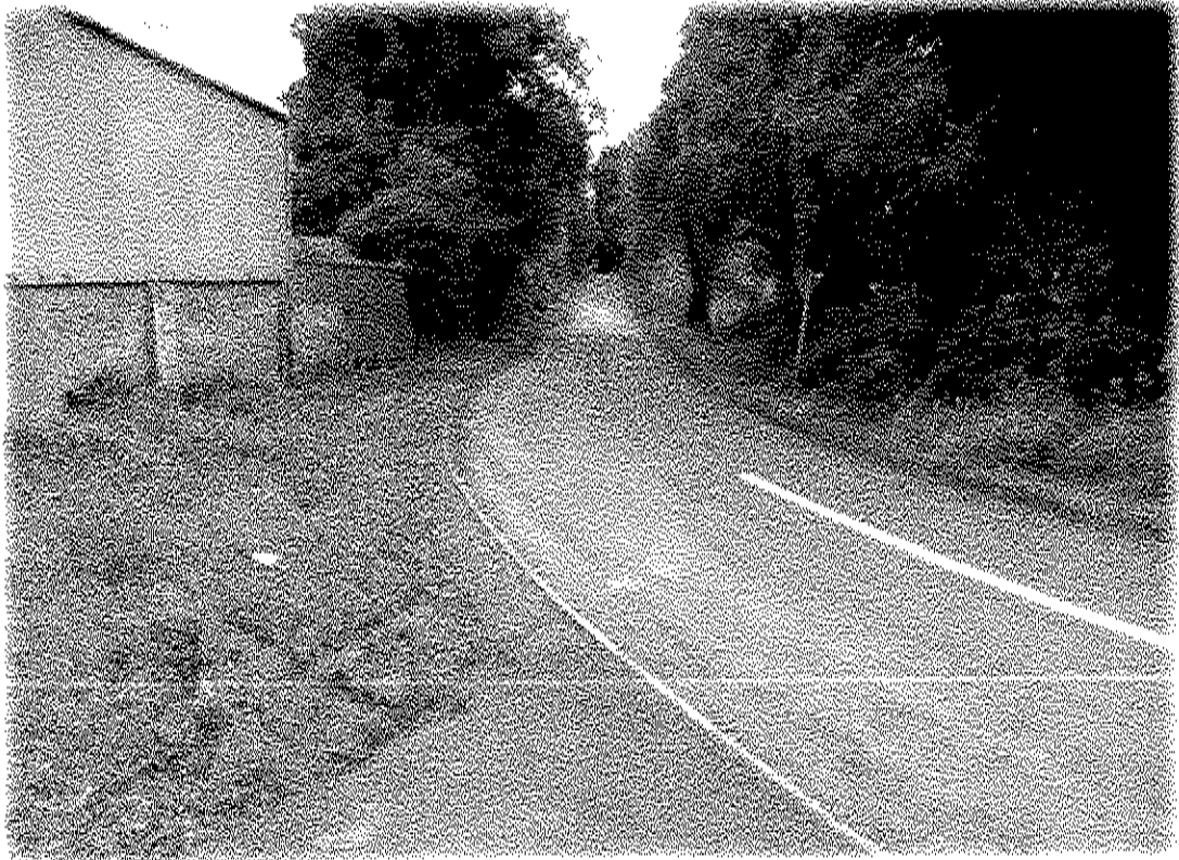
Footpath at Rushbrook, Claremorris - Prior to works
