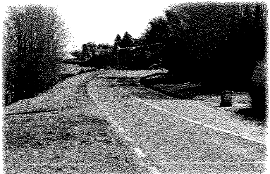
Completed pavement works
