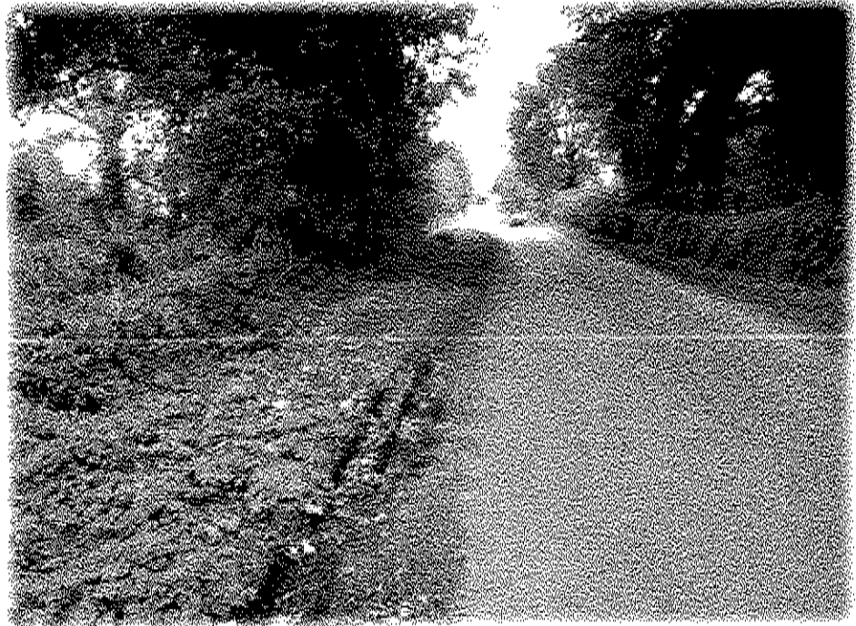
Footpath at Rushbrook, Claremorris Prior to works
