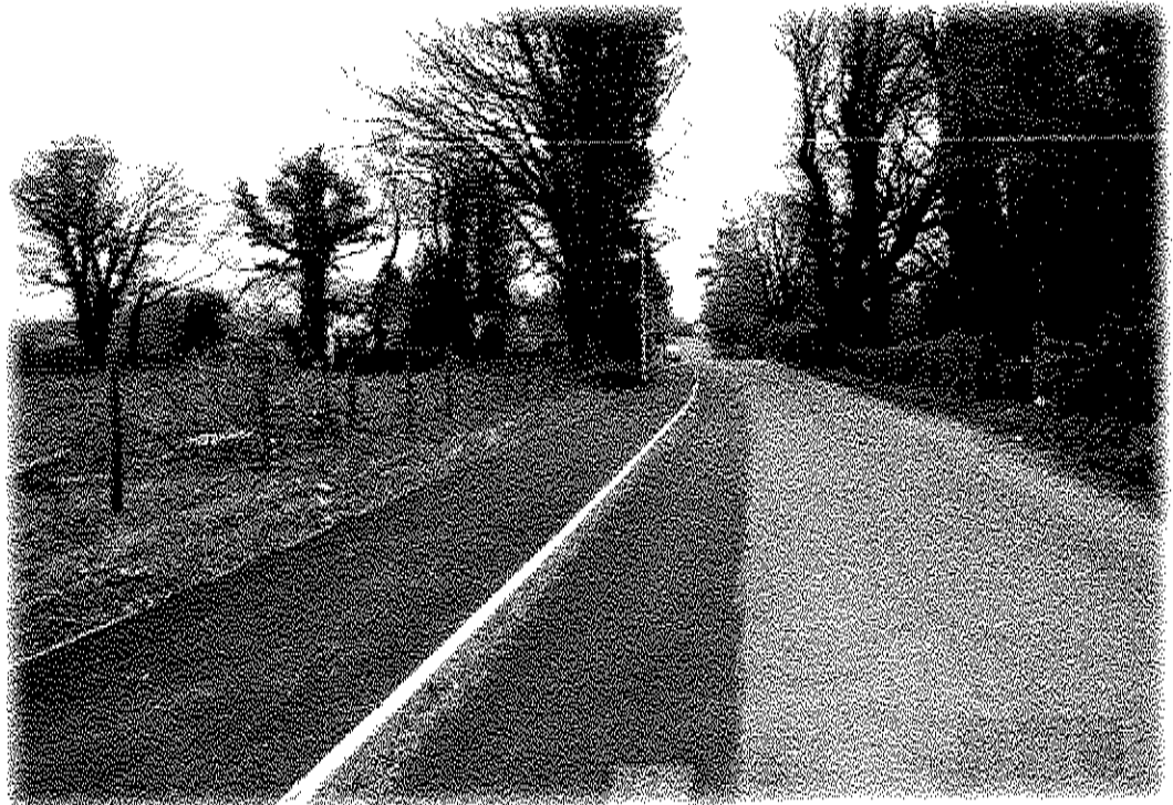
Footpath at Rushbrook, Claremorris Completed works
