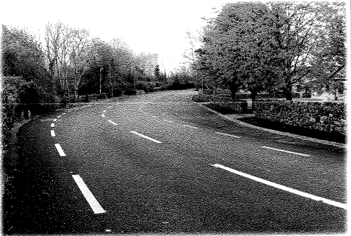
Completed pavement strengthening works at The Neale National School
