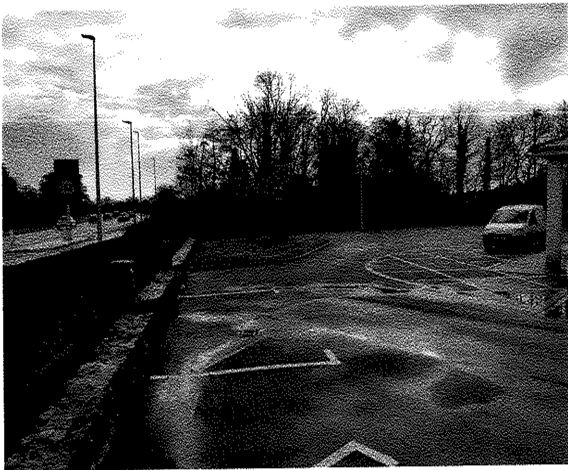
Bohola Car Park Extension
