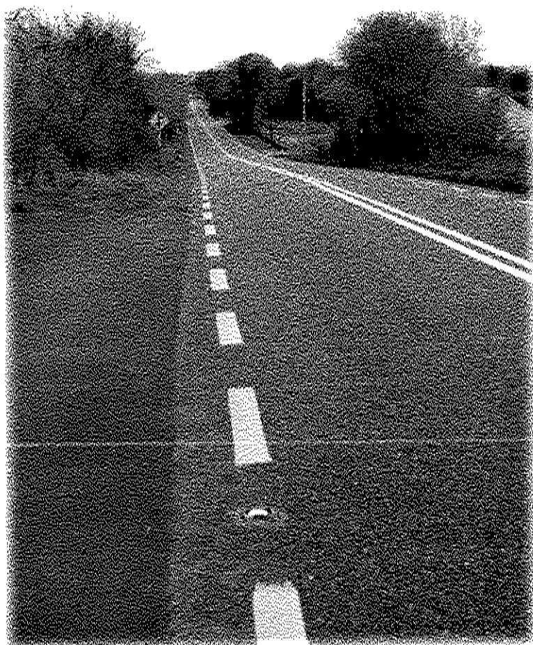
N60 Ballyhaunis / Ballinlough Road pavement strengthening works at Kiltybo
