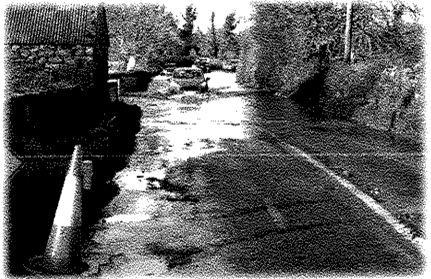
Flooding on the R334 at Dowagh
