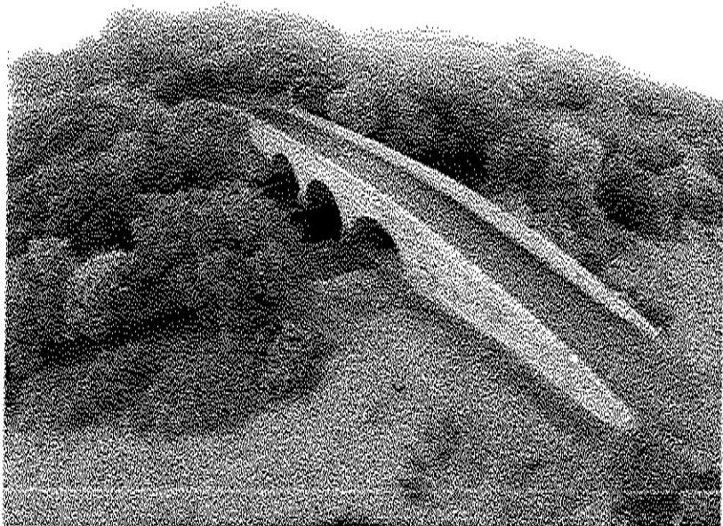
Richmond Bridge following restoration works
