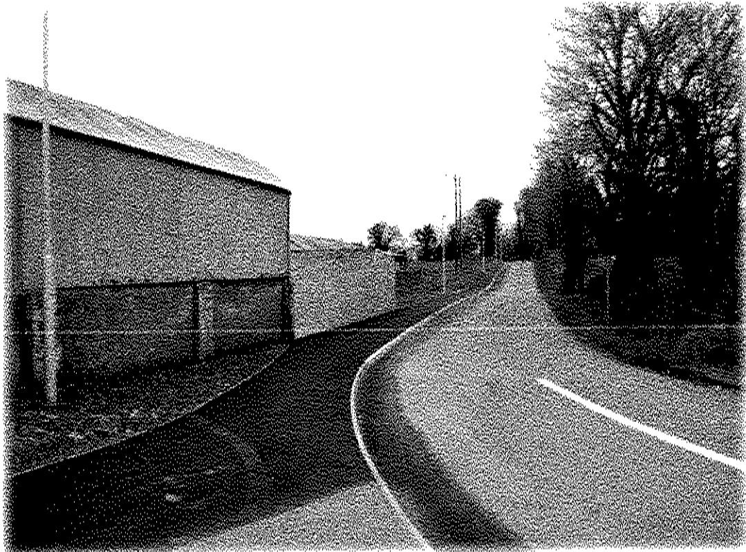
Footpath at Rushbrook, Claremorris - Completed works
