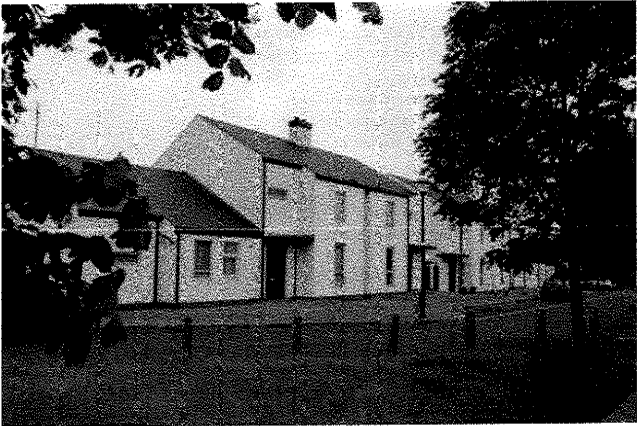
Ongoing local authority housing maintenance
