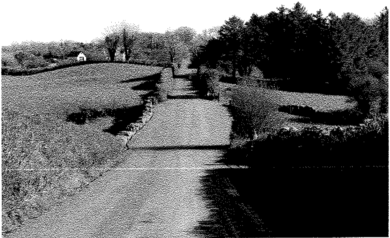
Remedial Works at Ballywalter
