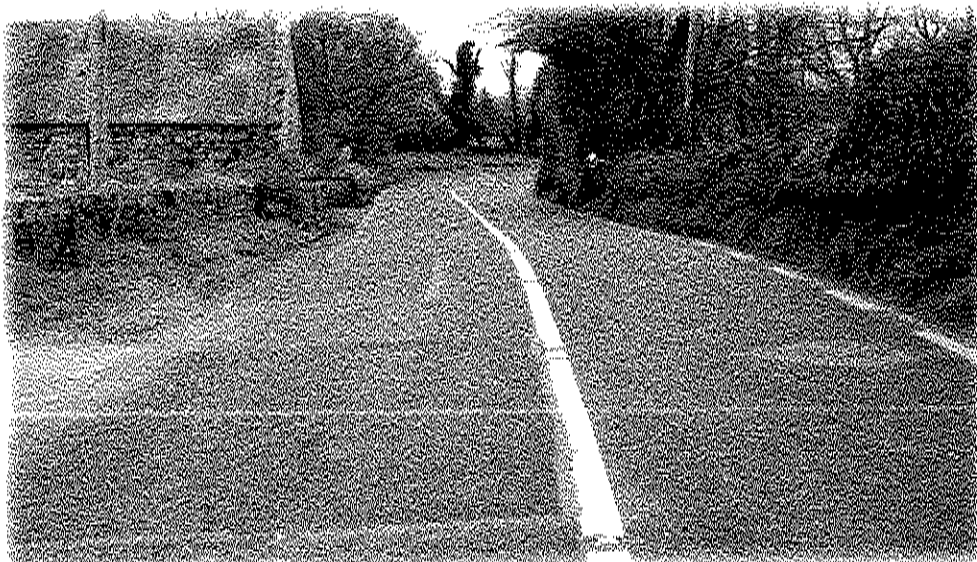
Completed pavement and drainage works on the R334 at Dowagh
