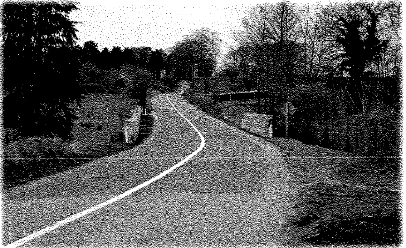
Tulrohaun Bridge, Claremorris—completed works
