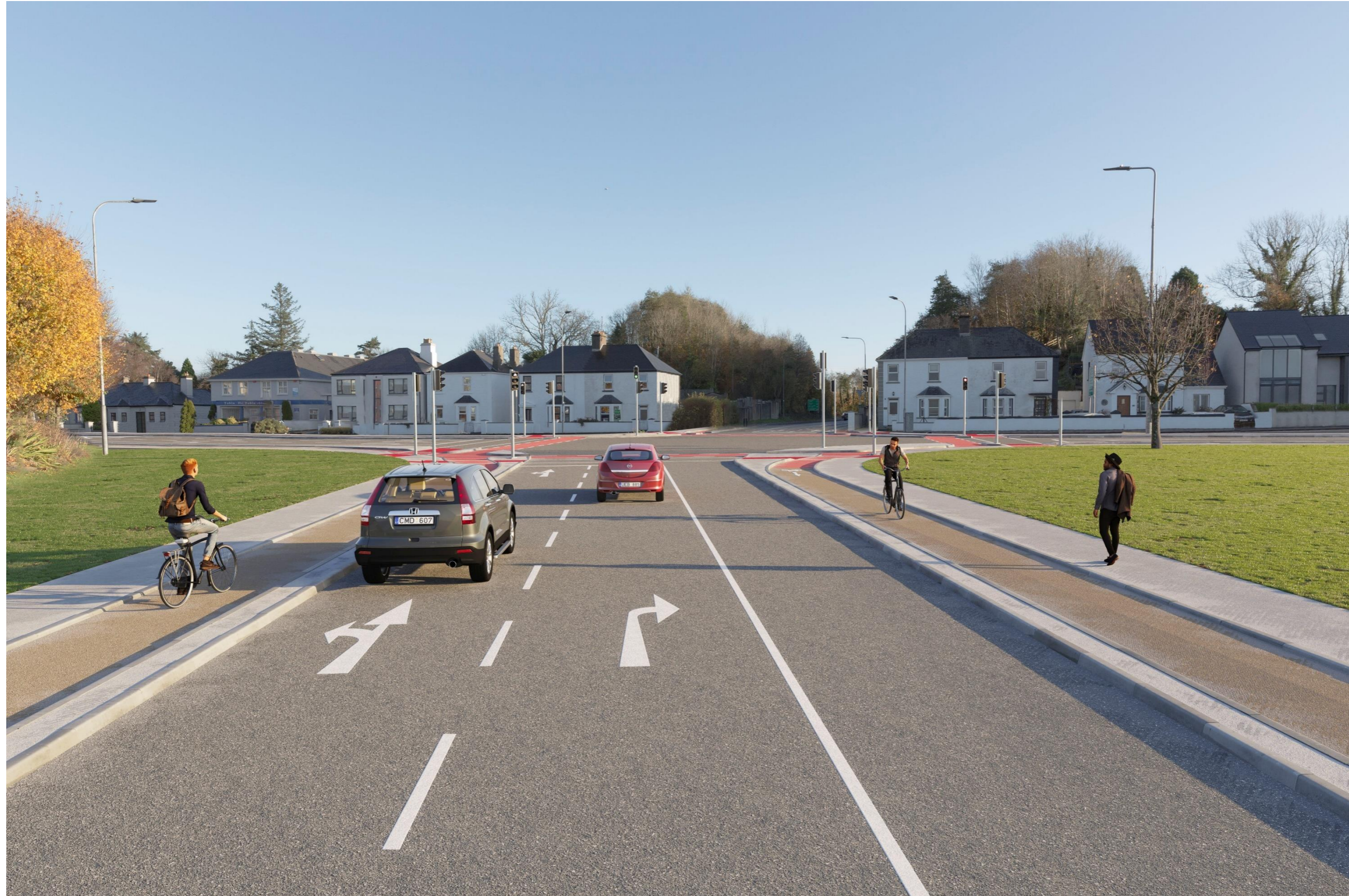
Figure 8-8: Draft layout of the proposed signalised junction along Station Road, Humbert Way, Spencer Street and Lawn Road viewed from Humbert Way
