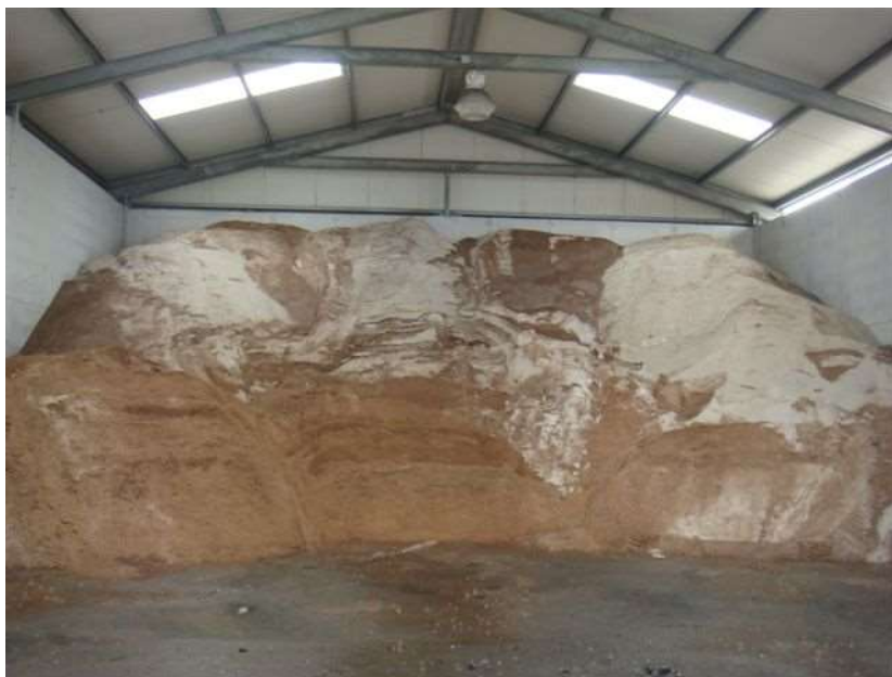
Figure 2: Salt storage barn
