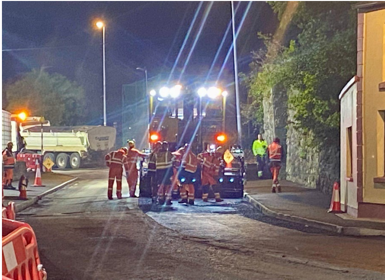
N59 George's Street Newport – Pedestrian Crossing Works
