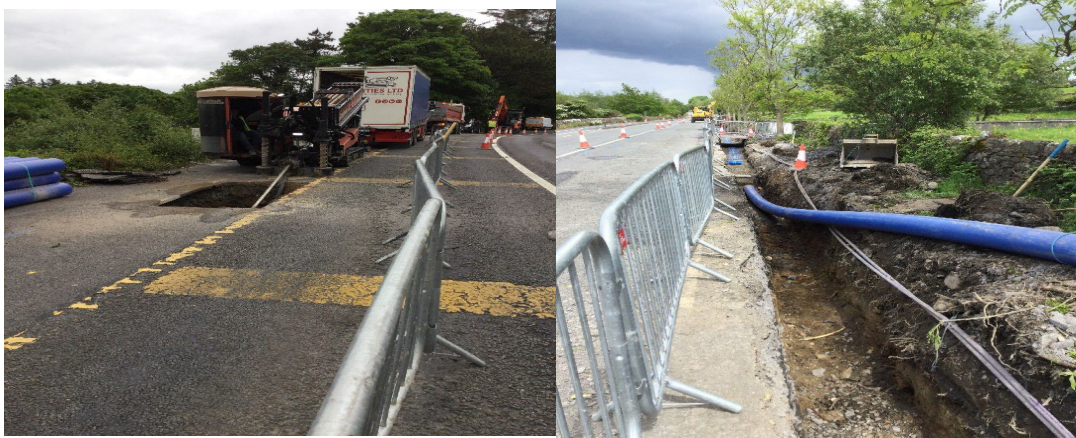
Construction works ongoing at Murrisk CWC
